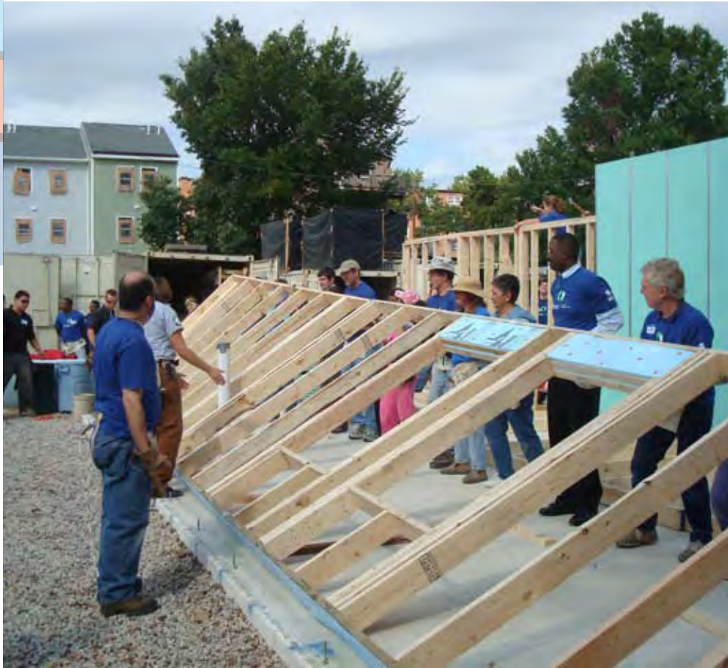
DC Habitat volunteers at work on Northeast Parcel development
