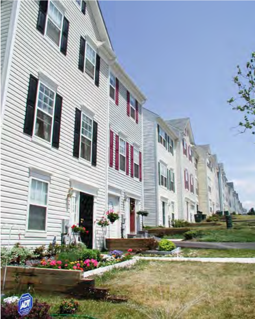
The Townhomes at Oxon Creek built by William C. Smith & Co.
